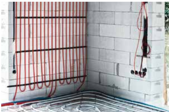
Wall or ceiling installation
